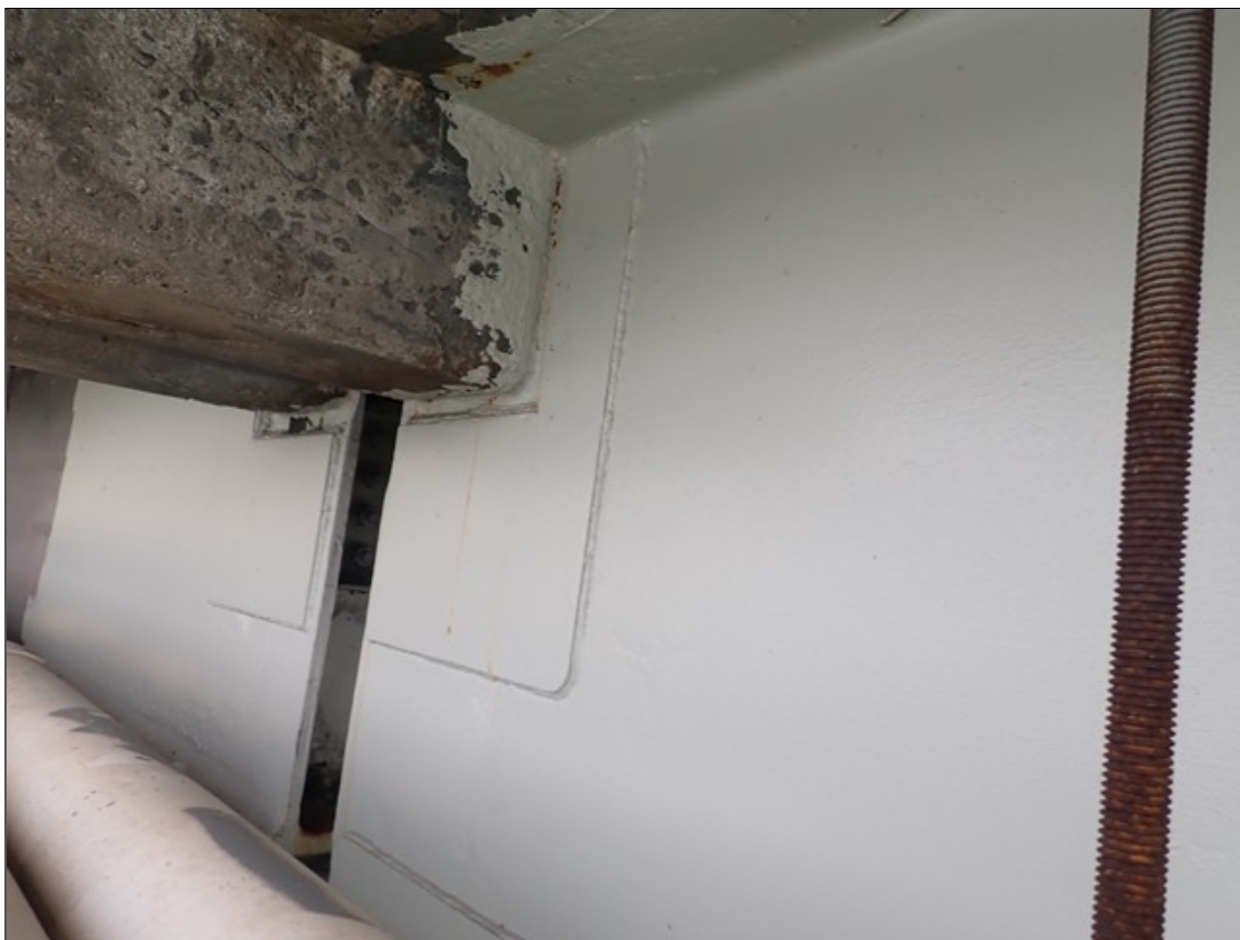
EXTERIOR BEAM 1 REPAIR PLATE AT BENT 9
