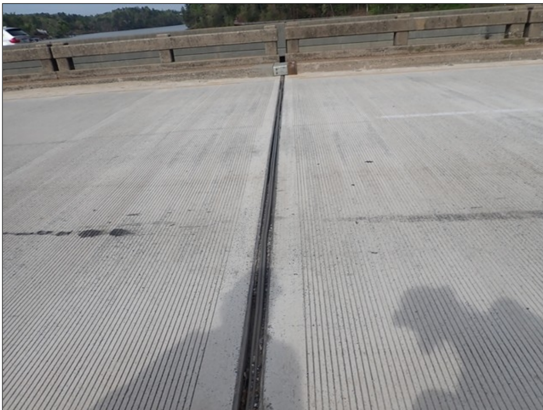
JOINT OVER BENT 5
