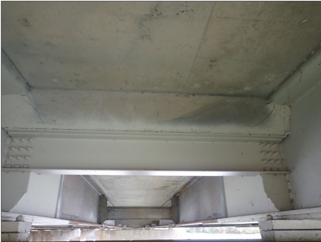
END DIAPHRAGM AT BENT 8
