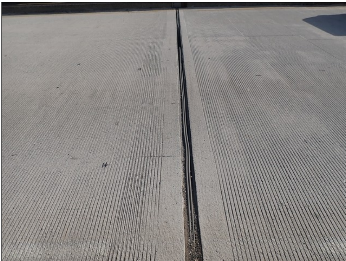
JOINT OVER BENT 9
