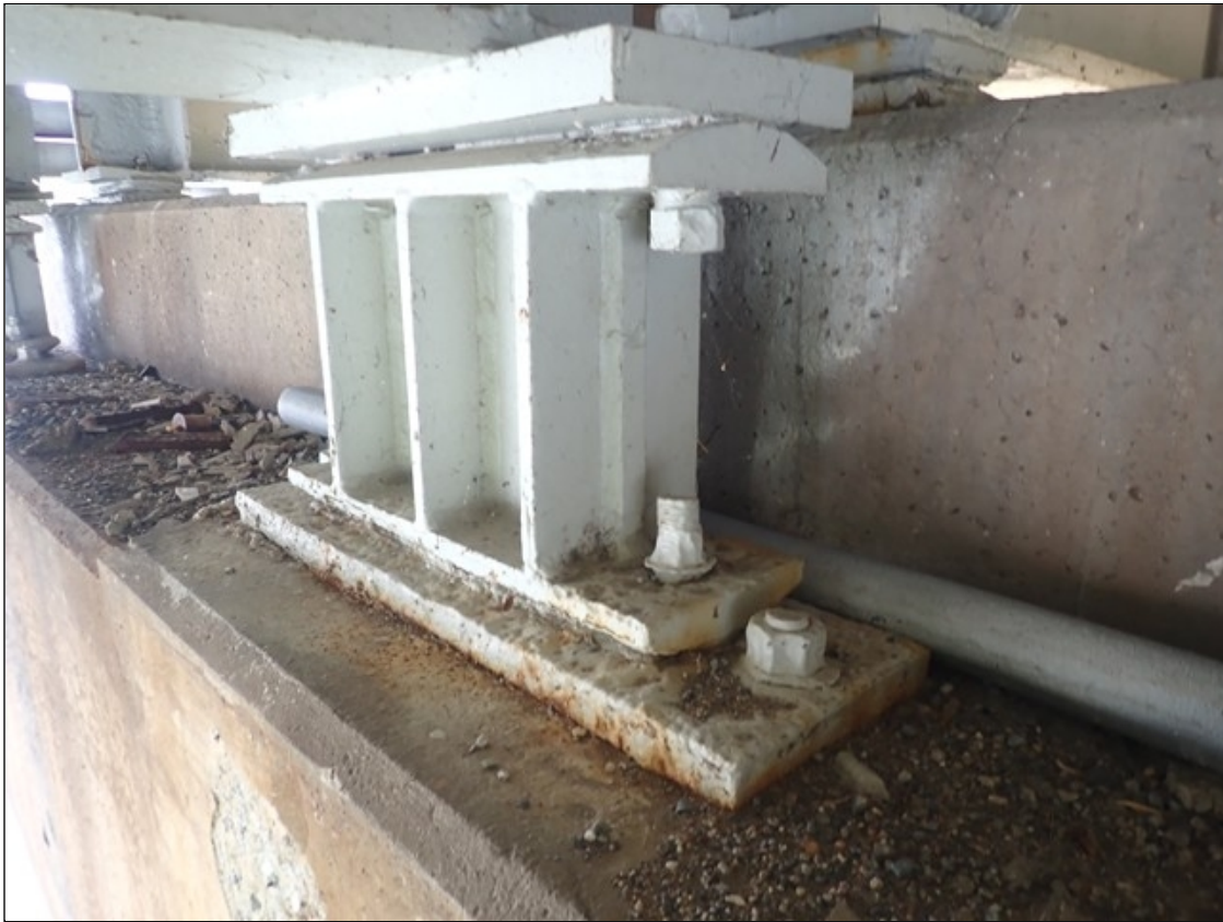
Span 6 Beam 2 Far Bearing - Protective System: SUBSTANTIALLY EFFECTIVE (CLEANED AND PAINTED)
