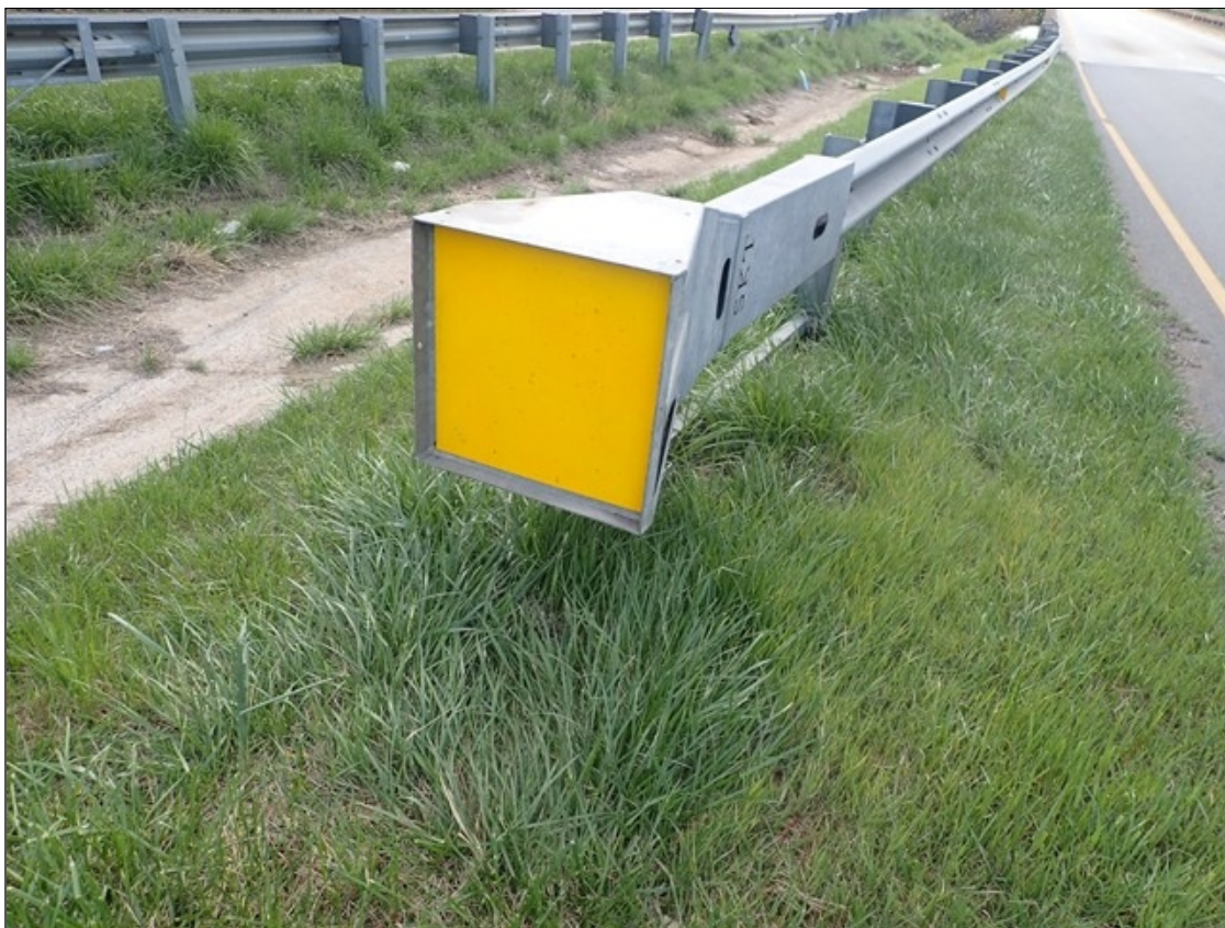
NORTHEAST GUARDRAIL TERMINAL
