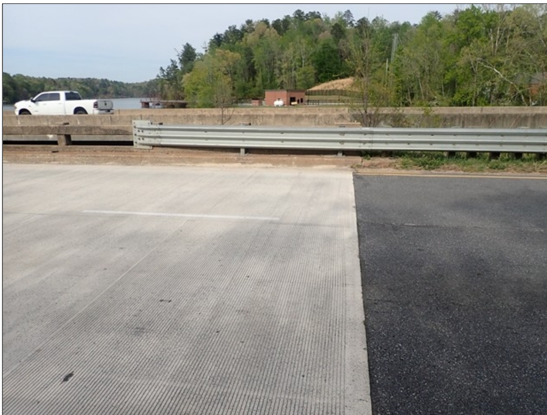
SOUTHEAST GUARDRAIL ATTACHMENT
