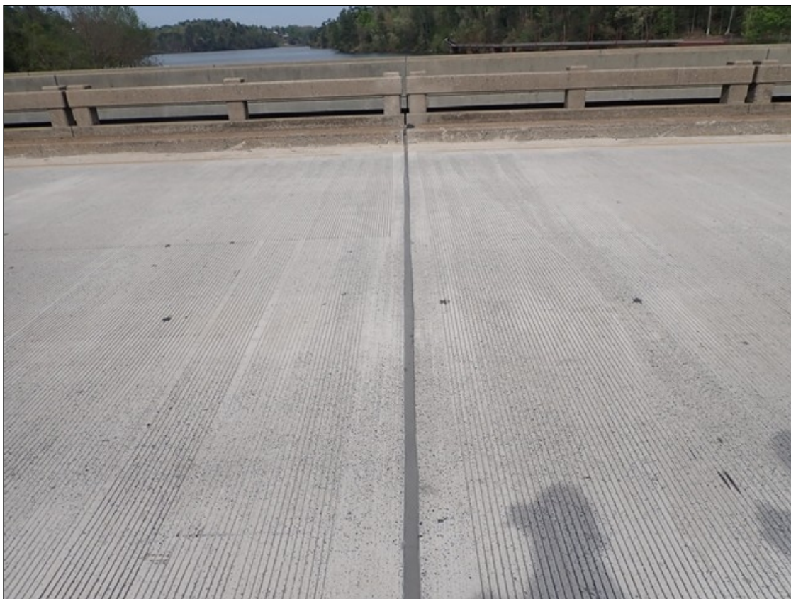
JOINT OVER BENT 8
