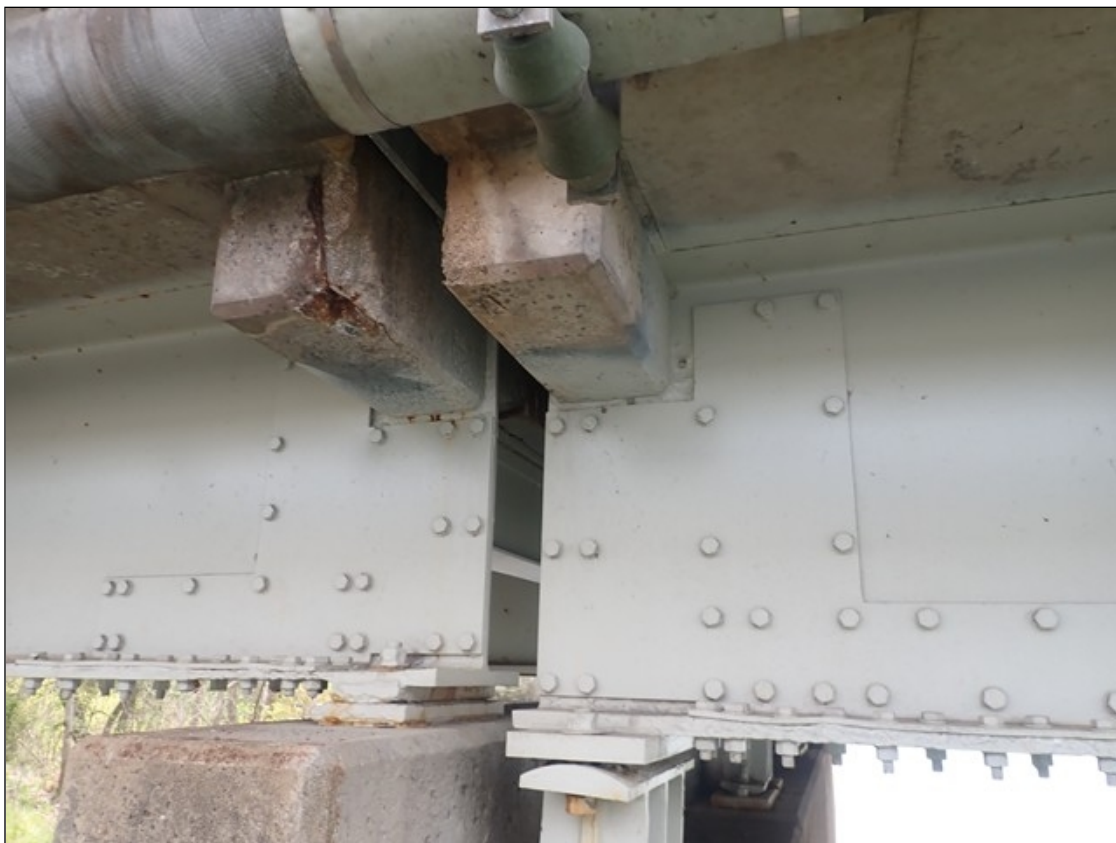
BEAM REPAIRS TO BEAM 4
