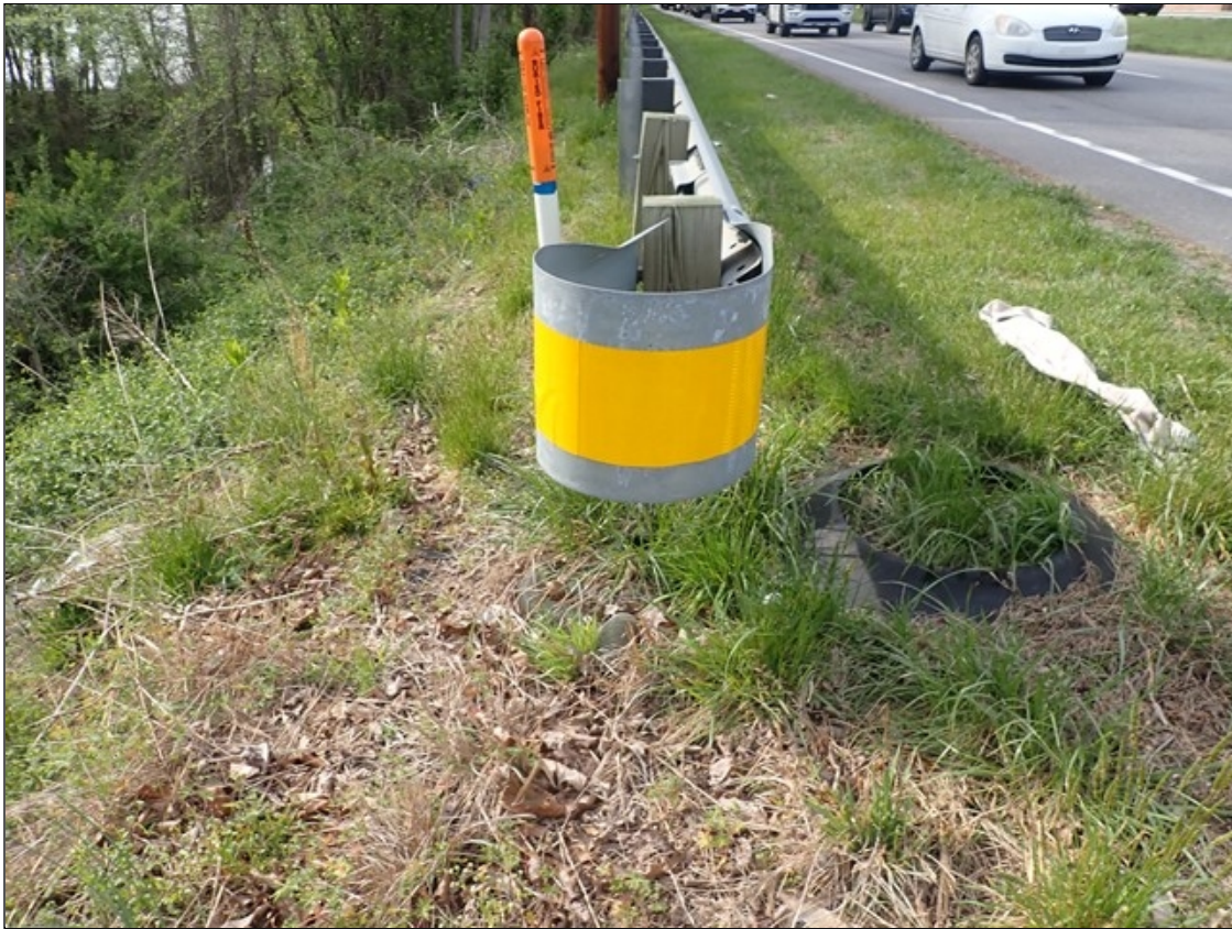
SOUTHWEST GUARDRAIL TERMINAL
