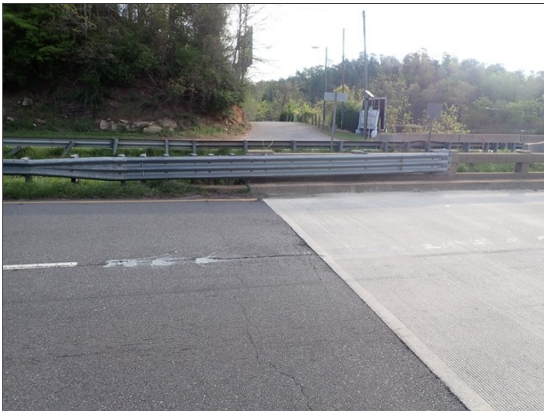
NORTHEAST GUARDRAIL ATTACHMENT
