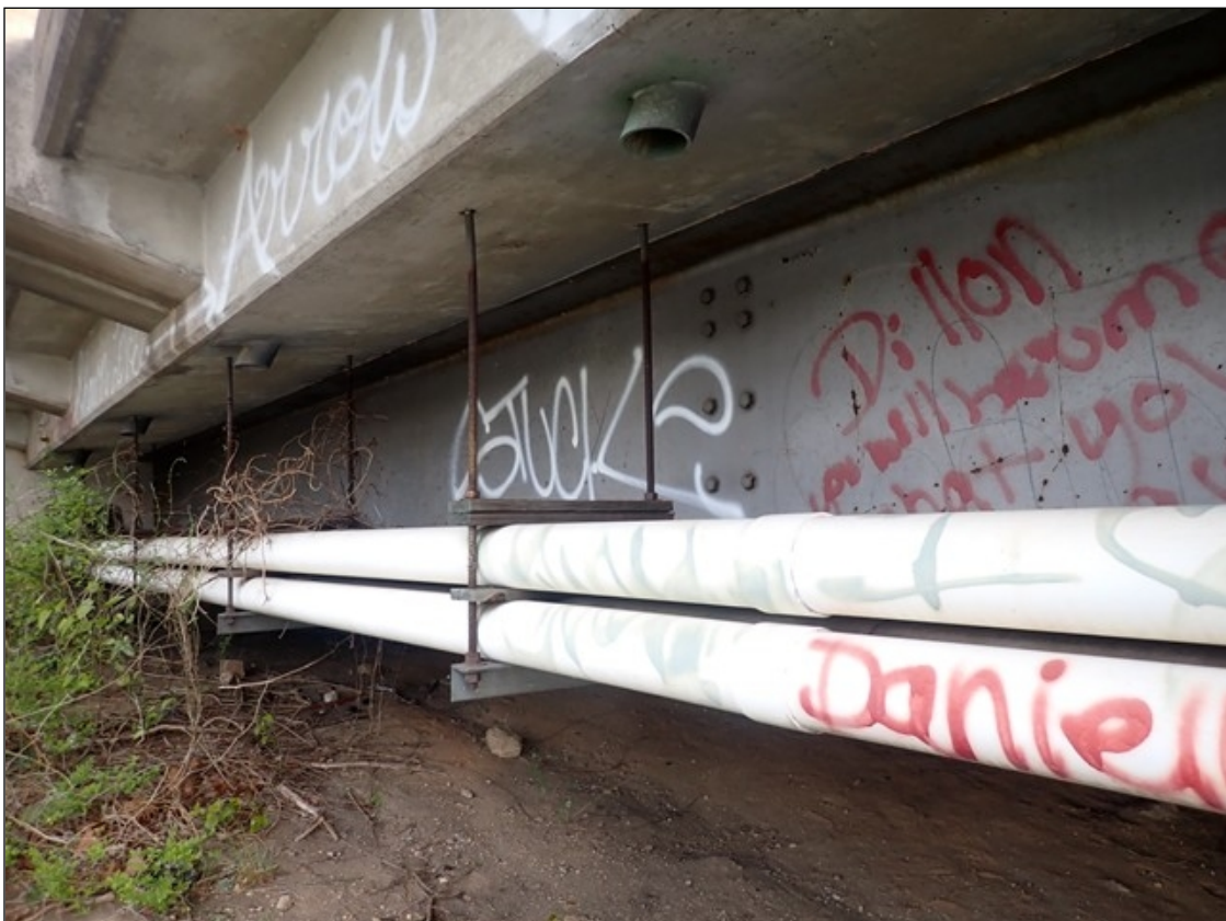
UTILITY WEST SIDE
