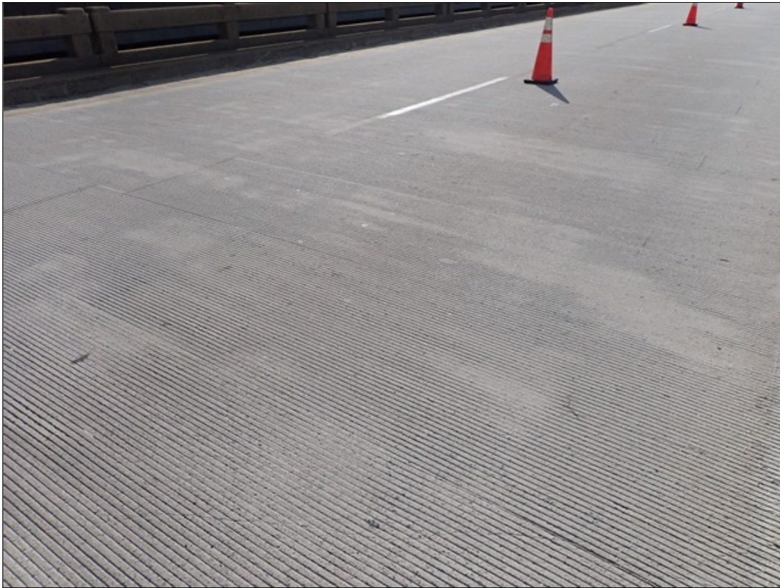
CONCRETE BRIDGE DECK
