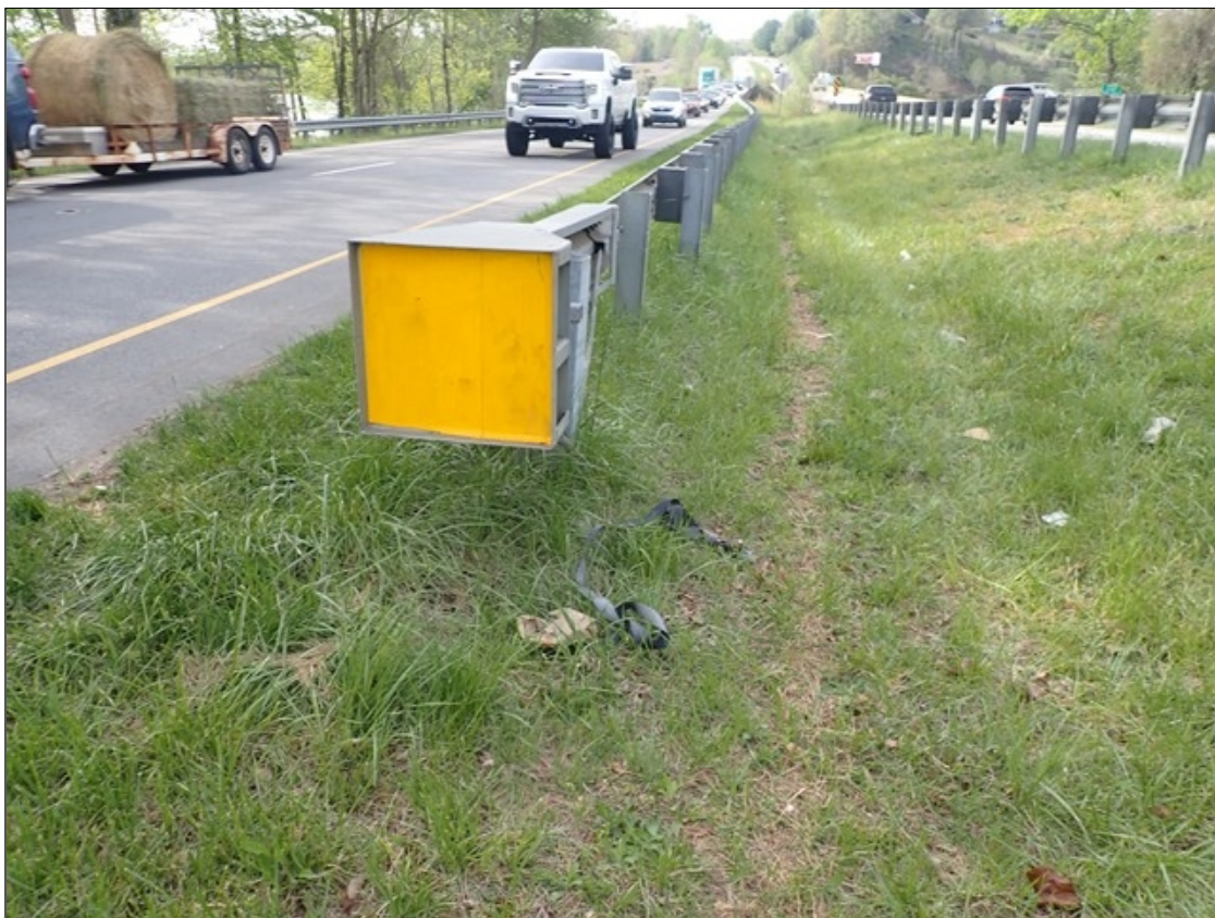
SOUTHEAST GUARDRAIL TERMINAL
