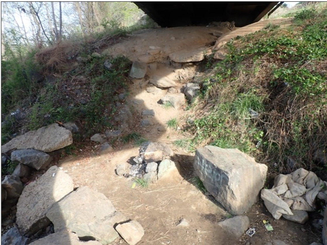
END BENT 2 SLOPE PROTECTION
