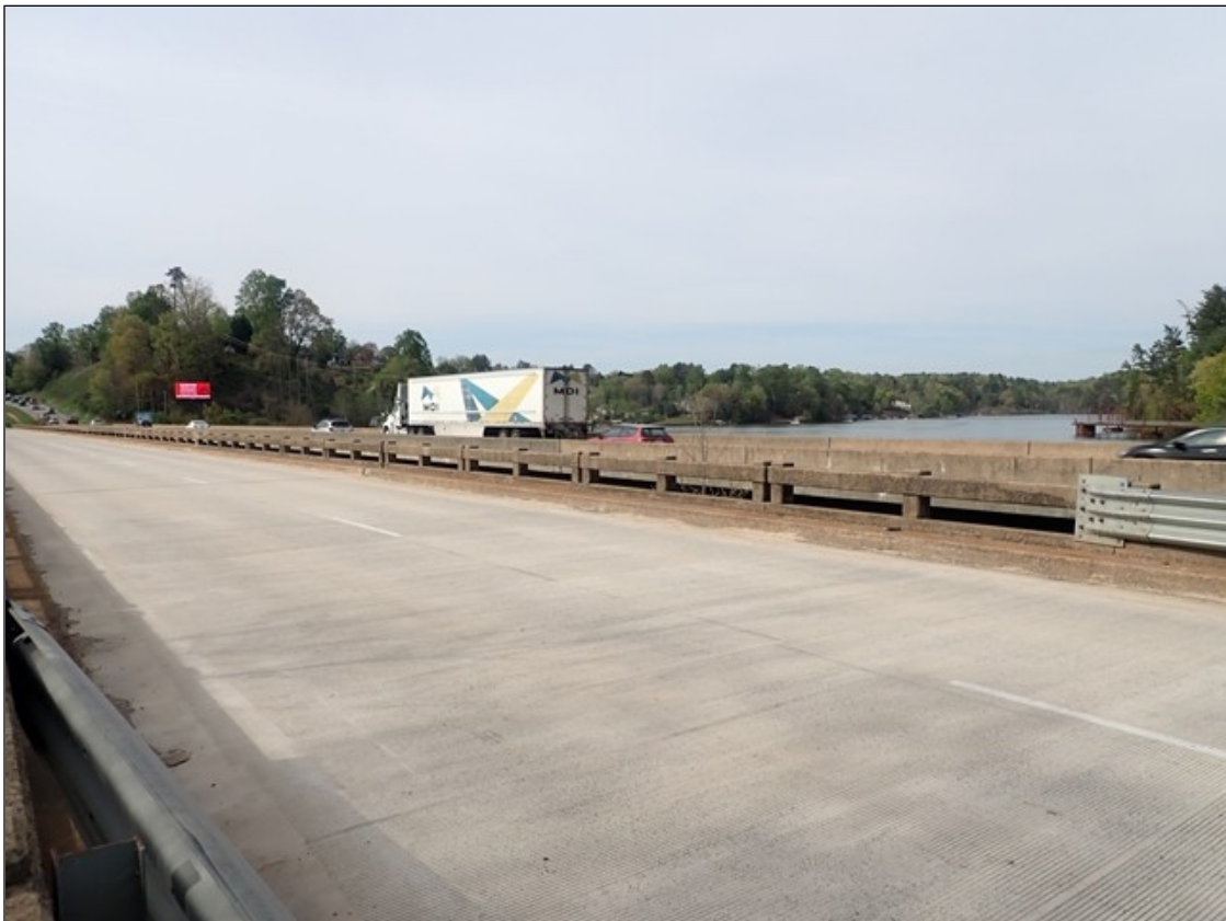
RIGHT BRIDGE RAIL
