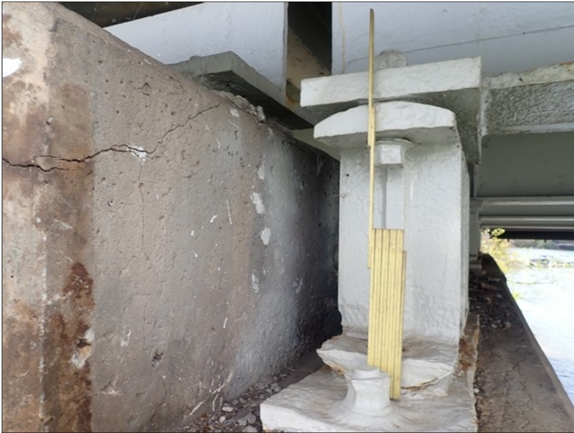
Span 6 Beam 1 Far Bearing - Protective System: SUBSTANTIALLY EFFECTIVE
