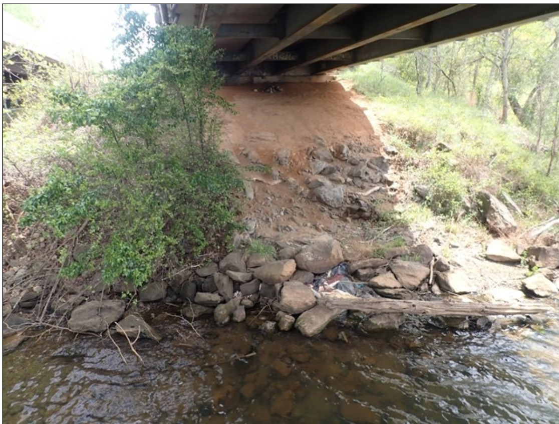
END BENT 1 SLOPE PROTECTION
